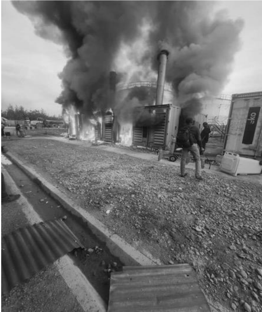
Photograph depicting burning generators at Twangiza mine, after the airstrike Confidential source
